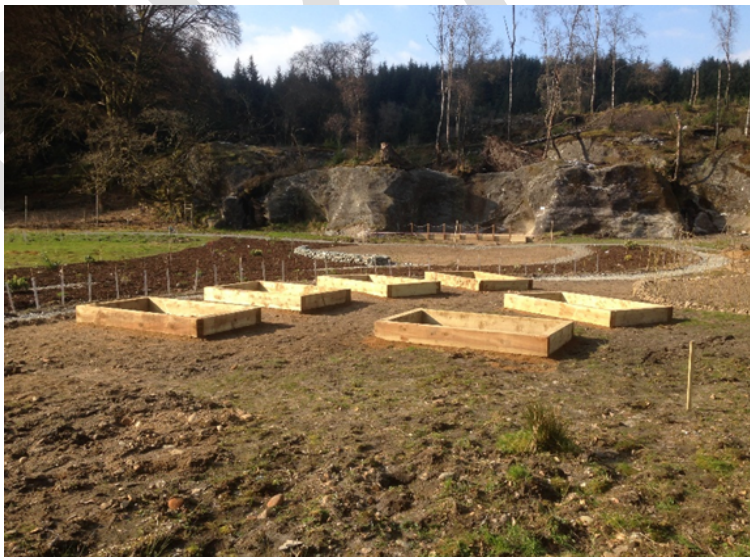
Lochgilphead Community Growing Space- construction phase.
